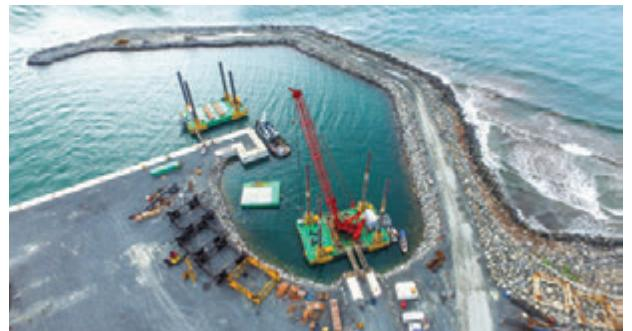
Jack up equipment with 400 ton capacity with 300 ton capacity crane over deck.
