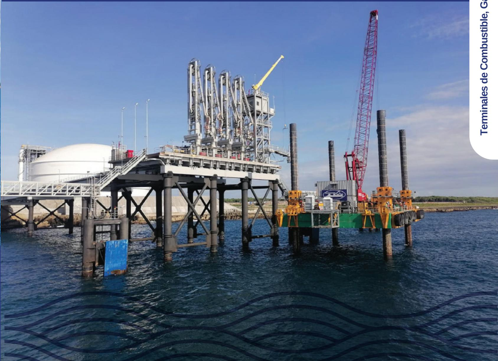
Supply of materials, equipment and labor for the reinforcement of 6 mooring dolphins and the installation of 10 new quick release hooks (QRH) for the AES ANDRES LNG terminal, located in Santo Domingo, Dominican Republic.
